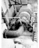
Figure 2: Francis turbine in La Herradura plant (EPM)
