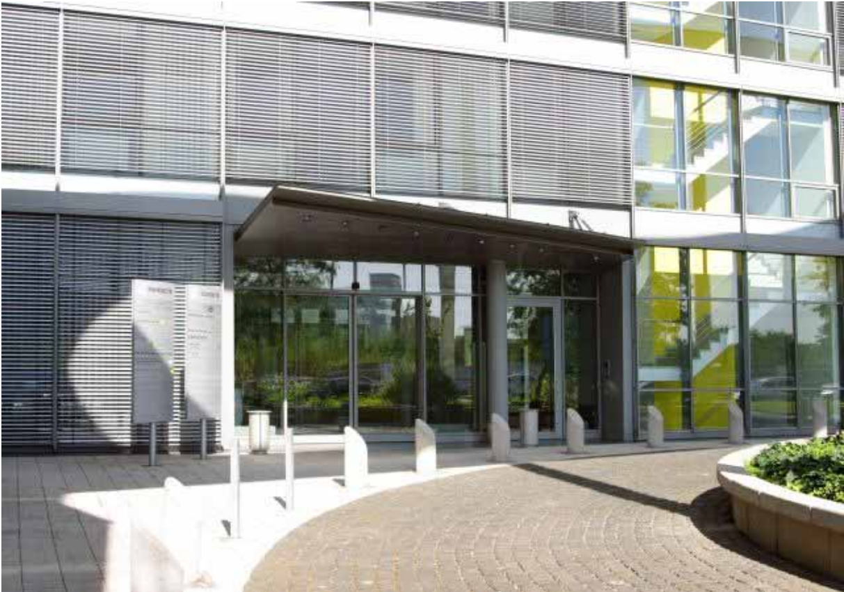
Image 2: Entrance of the Building
